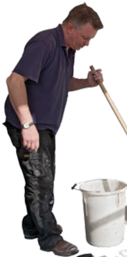
STOPGAP 1100 Gypsum being applied to STOPGAP P121 Acrylic Primer on a Calcium Sulphate screed
