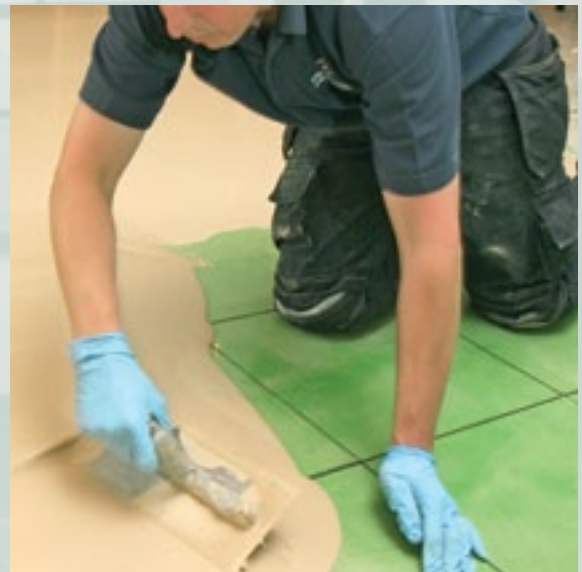
Applying STOPGAP 700 Superflex Fibre reinforced smoothing underlayment
