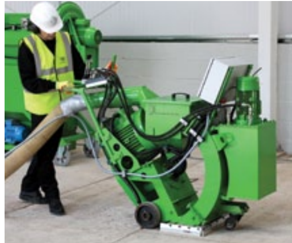
Shotblasting a floor with a vacuum dust free shot blaster
