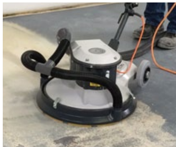
Grinding a floor
