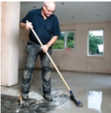
Use of a spiked roller to remove trapped air
