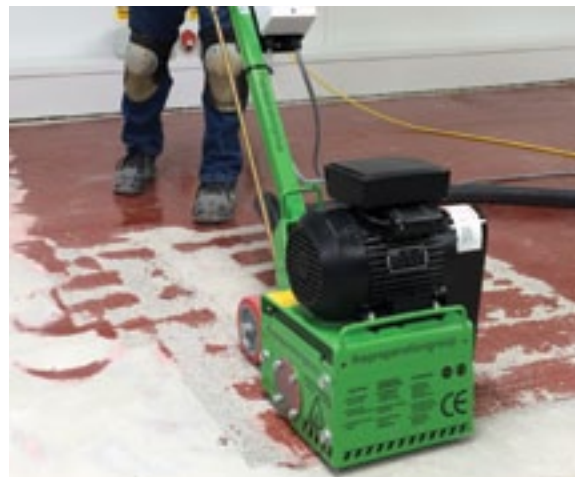
Using a mechanical planer
