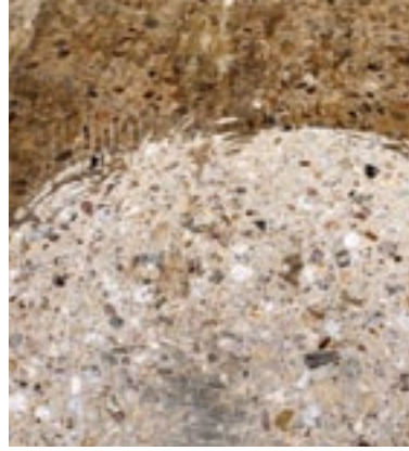
Adhesive residue removed by grinding
