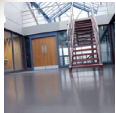
A floor prepared with WSM and underlayment prior to laying the finished floorcovering
