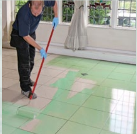
Applying STOPGAP P131 to an abraded ceramic tile floor
