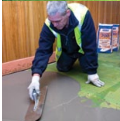
Applying STOPGAP 700 Superflex to a primed plywood floor
