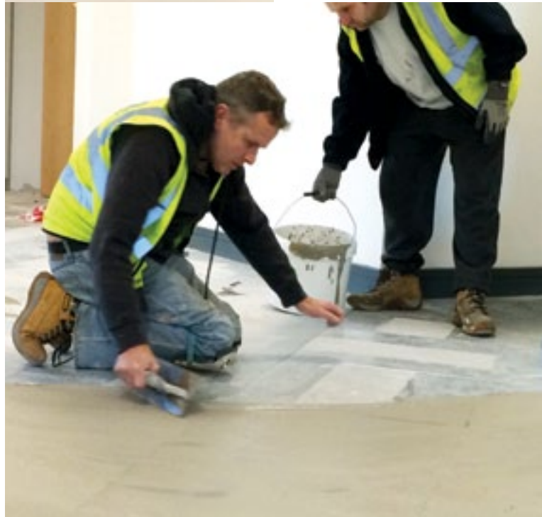
STOPGAP Fill & Prime applied to raised access floors prior to the application of an appropriate smoothing underlayment
