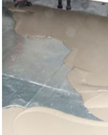
STOPGAP Fill & Prime applied to raised access floors prior to the application of an appropriate smoothing underlayment
