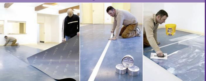
The Stopgap Isolator System was employed when low winter temperatures meant an extended drying out period for a newly laid sand/cement screed in a refurbished church hall. Use of the Isolator membrane, jointing tape and Styccobond F47 adhesive facilitated the rapid return to use of the building by enabling the flooring installation to be completed in 1½ days. This is in contrast to the 4-5 days a traditional two-coat liquid surface membrane and re-screeding would have required.
