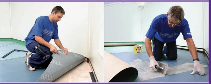
The Isolator system also dramatically reduced floorcovering installation time at Warwick Hospital where contractors were faced not only with a damp subfloor but also pressure to keep the job running. With the damp safely isolated by the membrane, specialist anti-bacterial linoleum was then bonded to it using Styccobond F84 all in sufficient time to meet the tight deadline.
